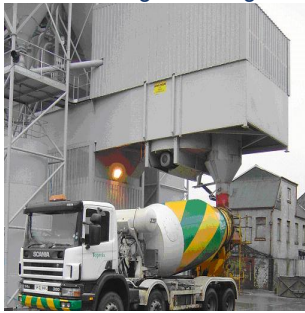
drive through loading point
