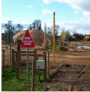
Public footpath flashing light system
