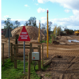
Public footpath flashing light system
