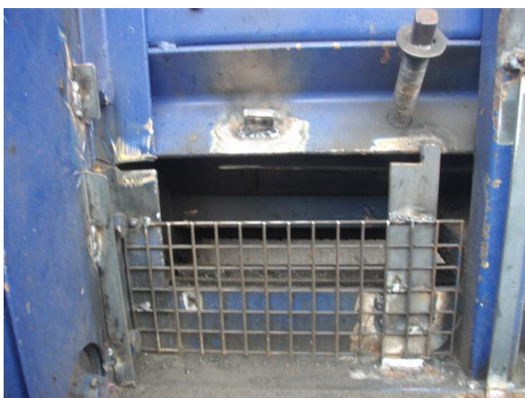
Brackets fitted to hold blanking plate
