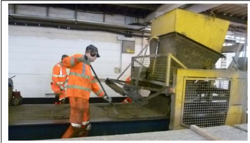
Figure 7.2 Wet casting T-beams
