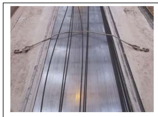
Figure 6.4 Wire restraint secured over hollowcore flooring bed.
