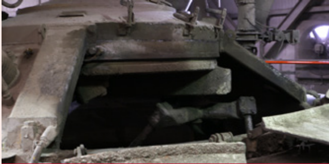
Entrance to mixer – confined space
