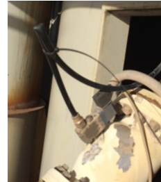
Above: this airline has been kinked to bypass the valve
